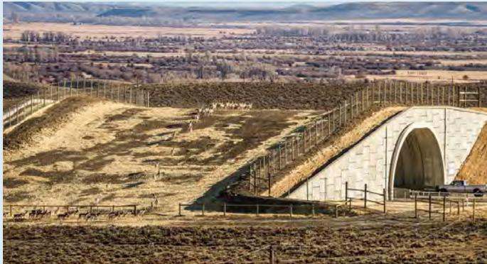
A **wildlife overcrossing** (left) is similar to a bridge or overpass and is designed to provide a seamless habitat connection over roads and railways. Effective overcrossings are vegetated and constructed to certain specifications regarding slopes and grades. They include directional fencing and design features to minimize noise from vehicular traffic.
