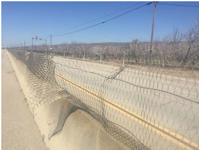
Figure 10. Picture of Monterey Road concrete median and wire fencing.
