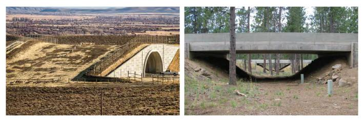
Examples of a wildlife overpass across Highway 191 in Wyoming (left) and a wildlife underpass under Highway 97 in Oregon (right).
