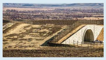
A wildlife overcrossing (left) is similar to a bridge or overpass and is designed to provide a seamless habitat connection over roads and railways. Effective overcrossings are vegetated and constructed to certain specifications regarding slopes and grades. They include directional fencing and design features to minimize noise from vehicular traffic.
