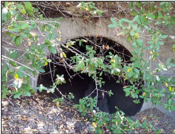
Photo 3. Culvert under Highway 101 at linkage number 10.
