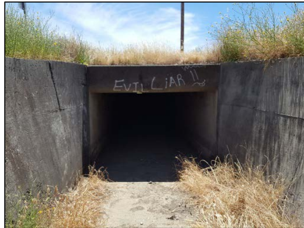
Photo 4. Culvert under Highway 101 at linkage number 11.
